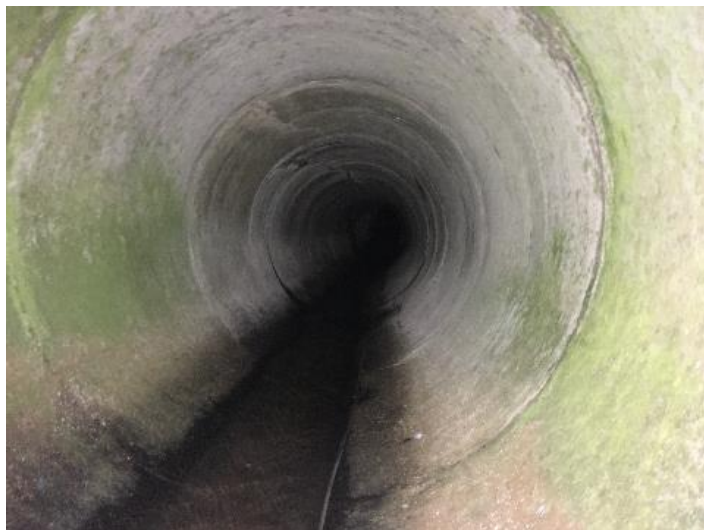
Watercrossing Structure W21
