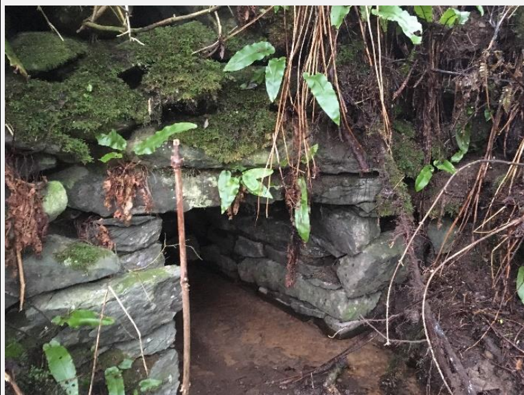
Watercrossing Structure W59
