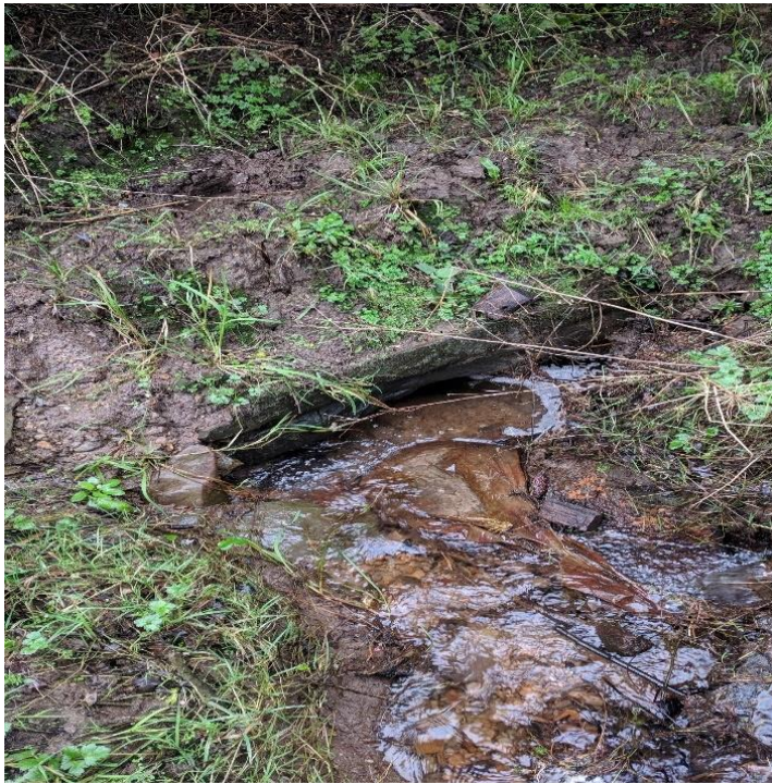
Watercrossing Structure W37
