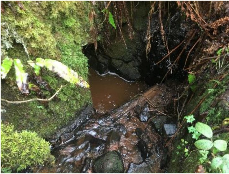
Watercrossing Structure W25
