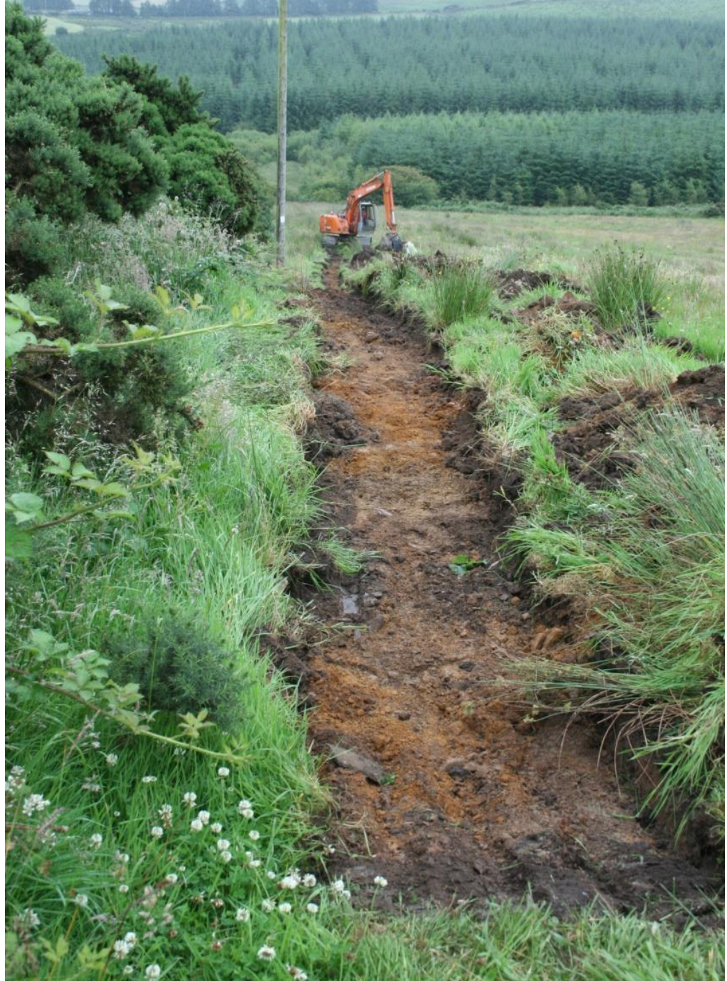
Figure 3: Test excavations underway, taken from west.
