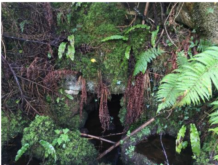
Watercrossing Structure W8
