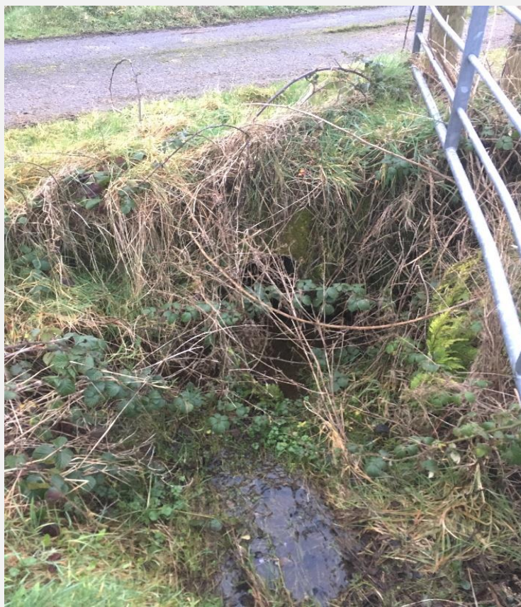
Watercrossing Structure W63
