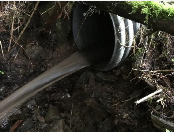
Watercrossing Structure W20
