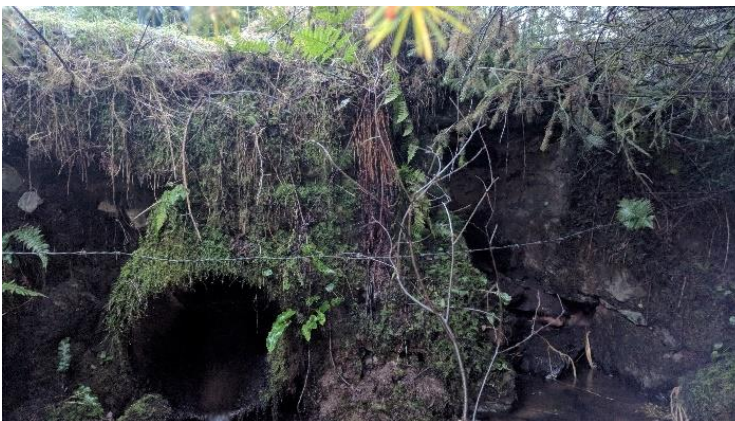
Watercrossing Structure W54
