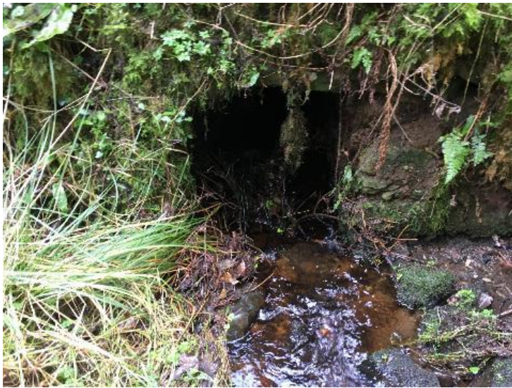
Watercrossing Structure W9
