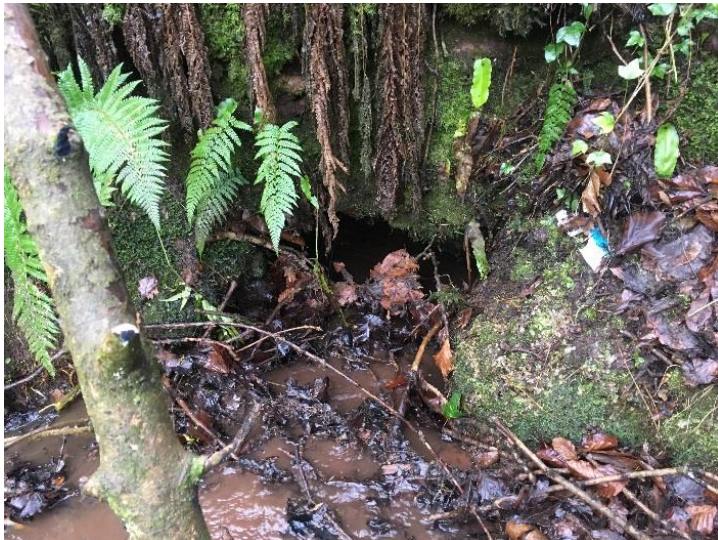
Watercrossing Structure W6
