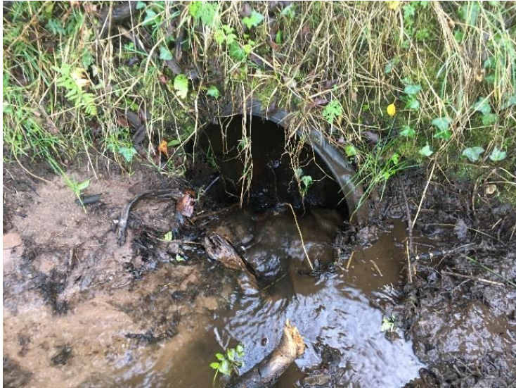
Watercrossing Structure W5
