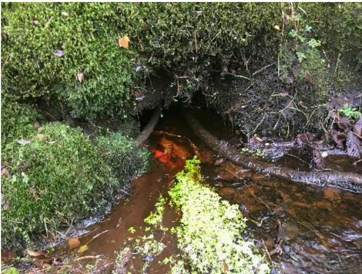
Watercrossing Structure W14
