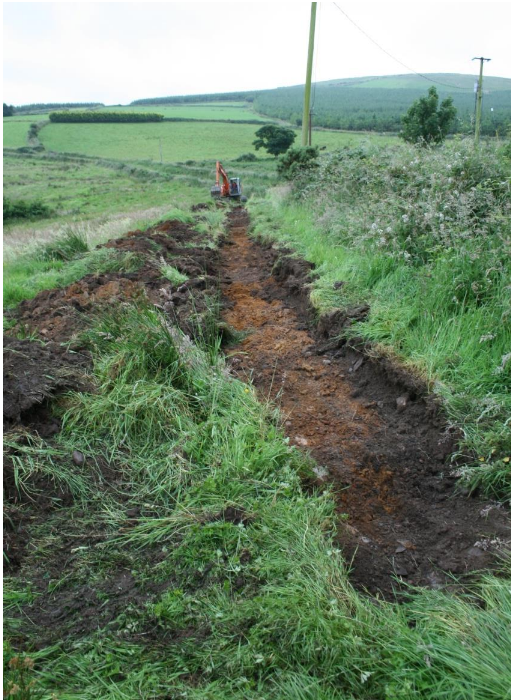
Figure 6: Trench 2 from the northeast
