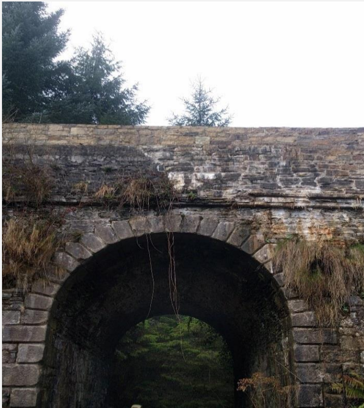
Watercrossing Structure W44
