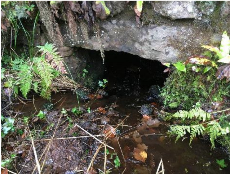
Watercrossing Structure W15
