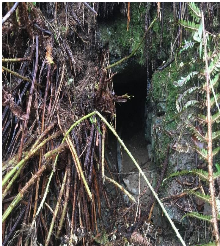
Watercrossing Structure W57
