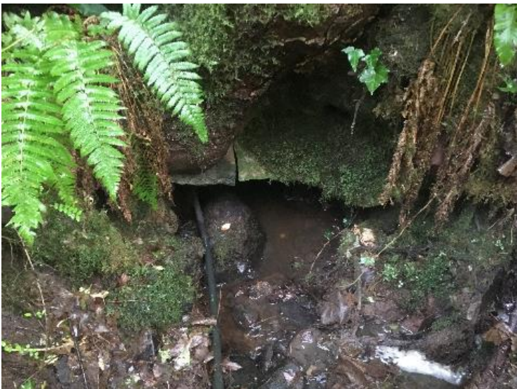
Watercrossing Structure W26
