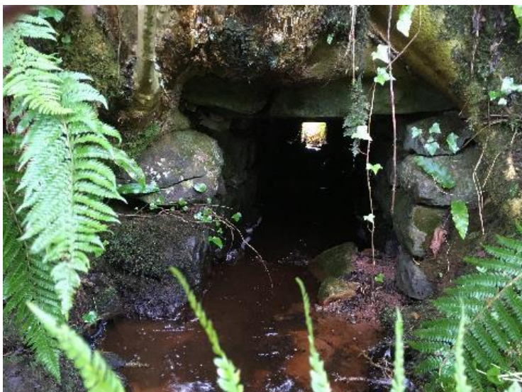
Watercrossing Structure W10
