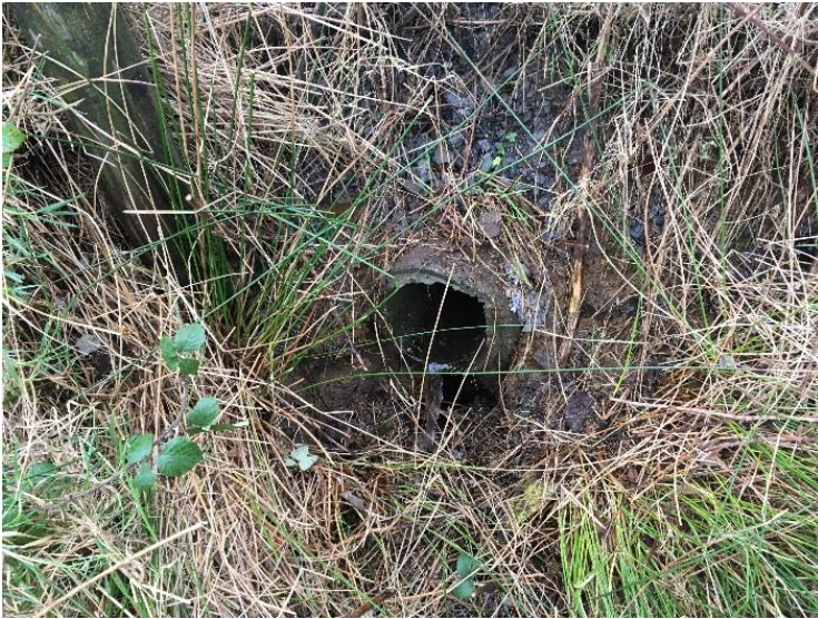
Watercrossing Structure W53
