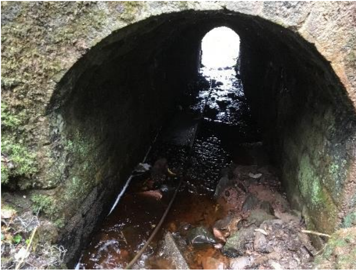
Watercrossing Structure W17
