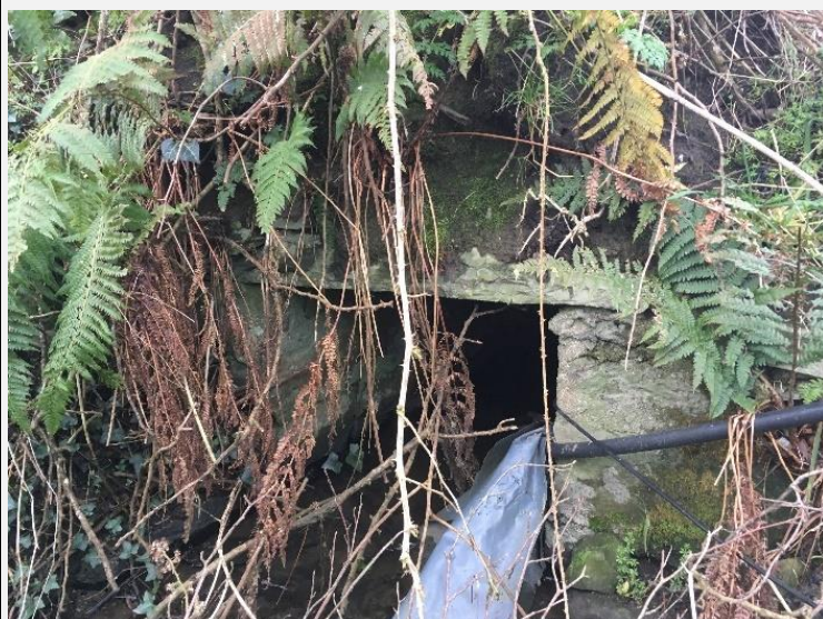
Watercrossing Structure W56
