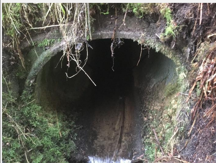
Watercrossing Structure W60
