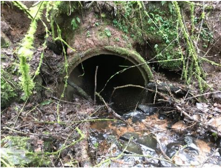
Watercrossing Structure W19
