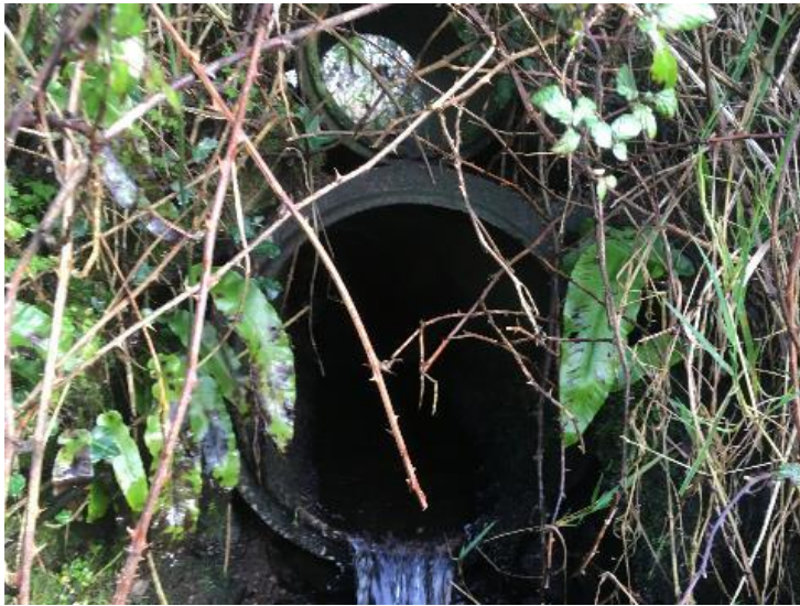
Watercrossing Structure W7
