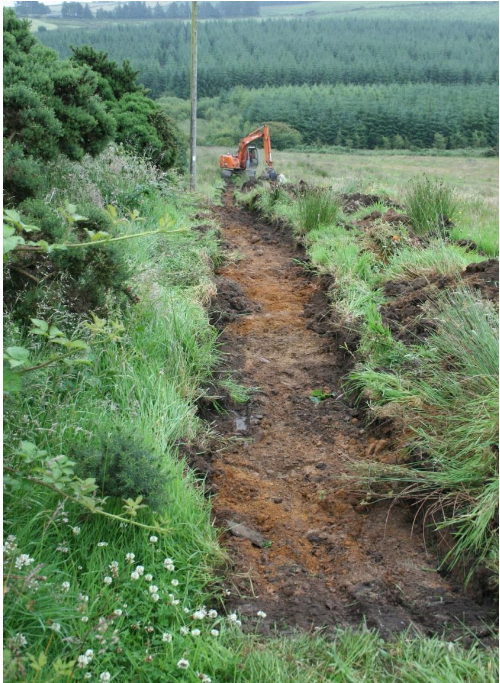
Figure 5: Trench 1 from the northeast
