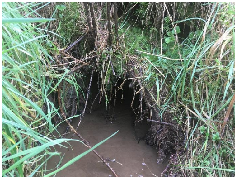
Watercrossing Structure W58
