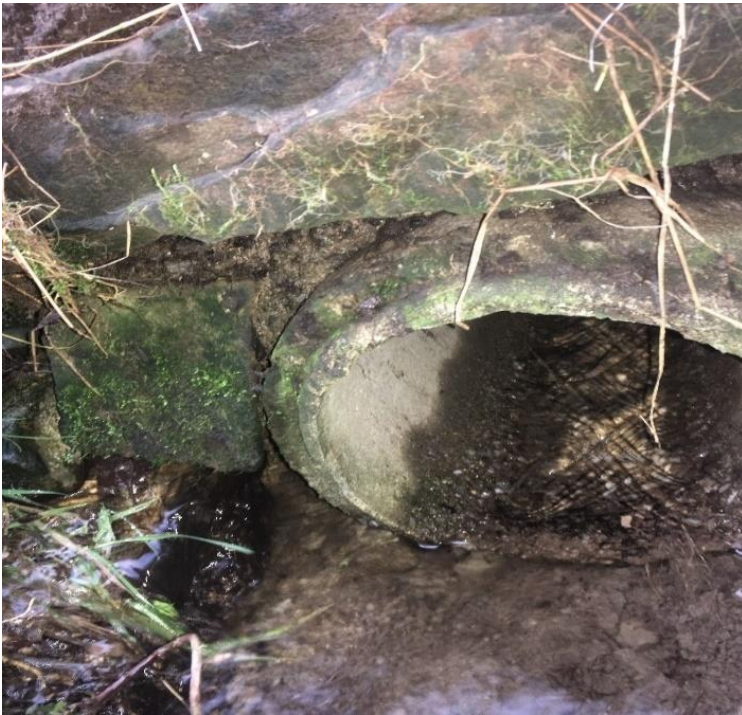
Watercrossing Structure W61
