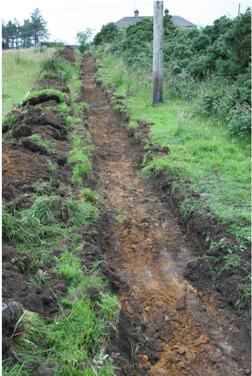
Figure 4: Trench 1 from the southeast
